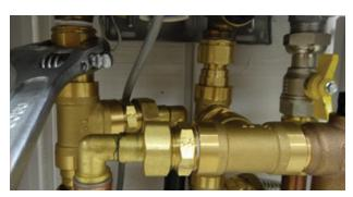
20 mm connector with spring-type non-return valve
